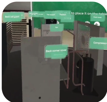
Exploded, labeled view of components with 360° turntable rotation.
